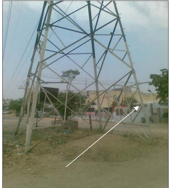
Coating Upto 3 Mtrs from Ground
