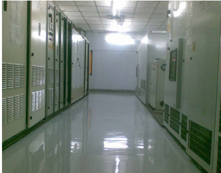
Panel Room Flooring
