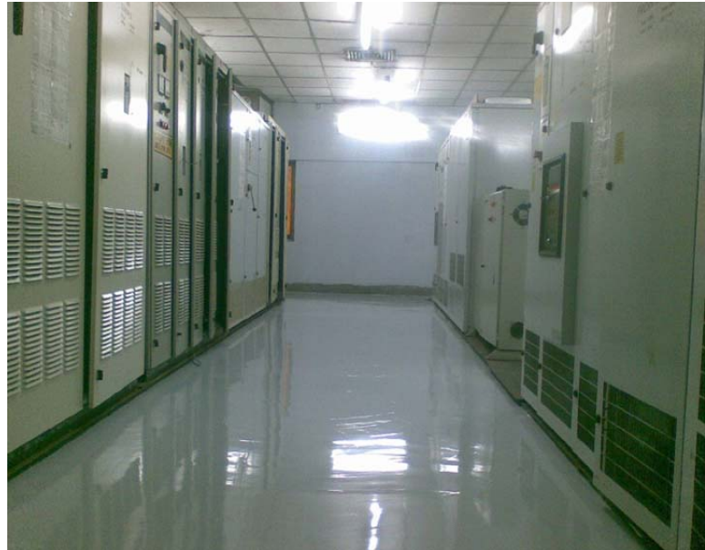
Panel Room Flooring
