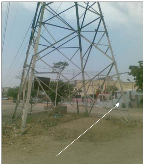
Coating Upto 3 Mtrs from Ground
