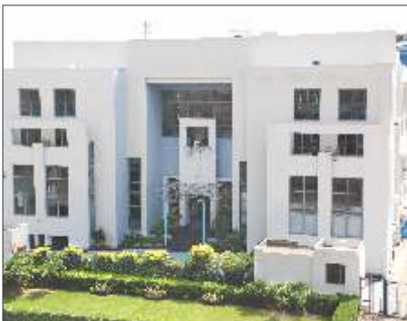
Plant -II, Manesar, Fabrication Welding Electrodes
