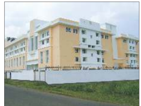
Plant -IV, Gurgaon, FCAW, Wear Plates...
